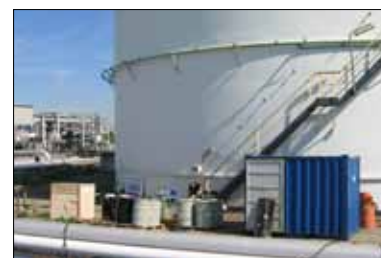
Tank lining in- and outside
