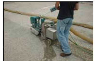
High pressure water blasting
