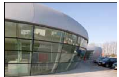
Roof- and facade finish
